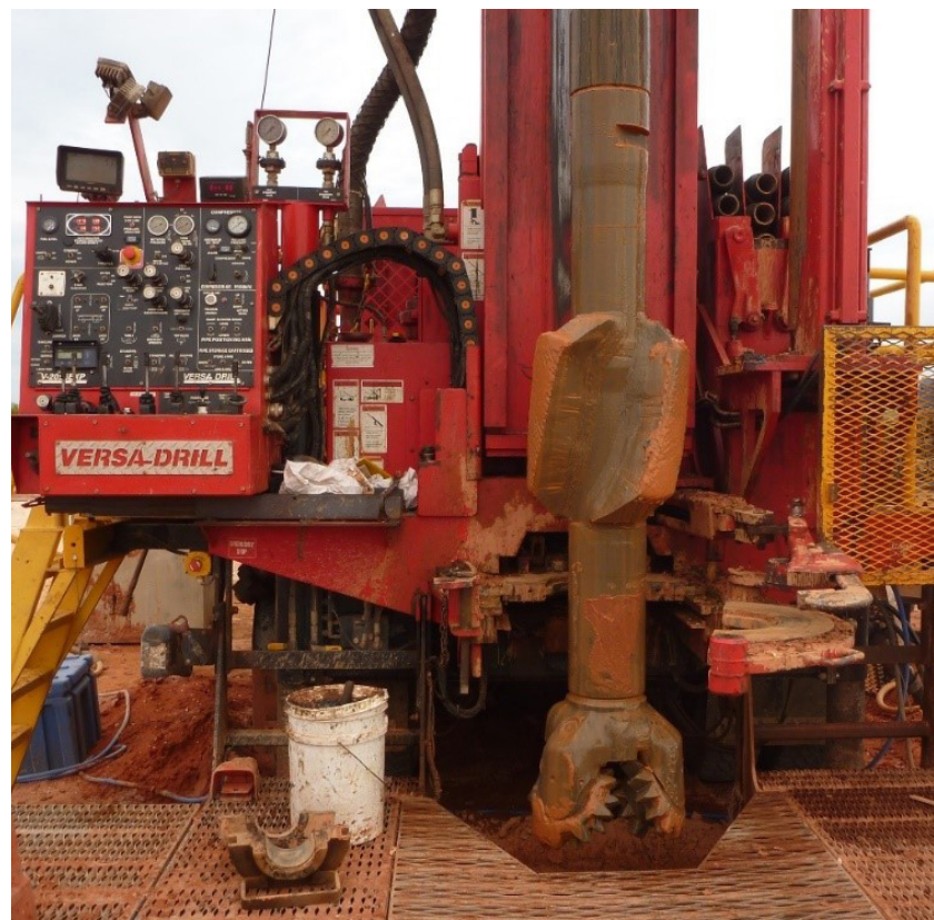
Rotary mud drilling Photo courtesy of Austral Drilling
